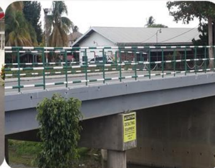
Mayfield Road Bridge
